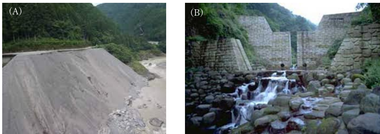
Figs. 6-5 Sediment movement countermeasures. (A) Deposited sand downstream of the Nagayasu Dam. Cited from Ministry of Land, Infrastructure and Transport. HP (B) Slit check dam. Cited from Ministry of Land, Infrastructure and Transport. Yuzawa sabo office. HP
