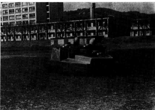
Fig. 3 Scorpion of amphibious two-seater craft provided bucket for reverse and braking. Complete hull structure is built in fibre-glass reinforced plastics. Maximum speed over land is 48km/h
